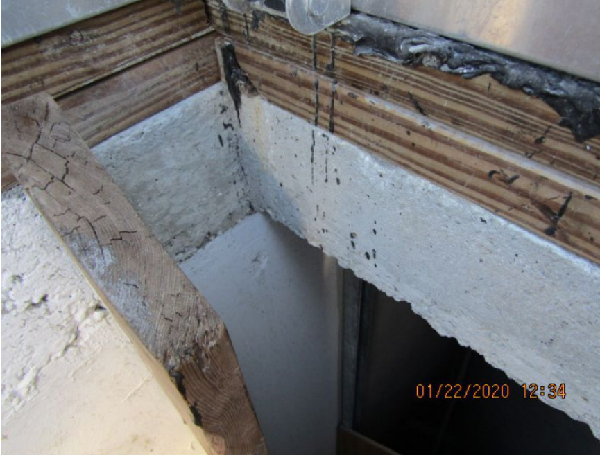
Reinforced Concrete Roof Deck
