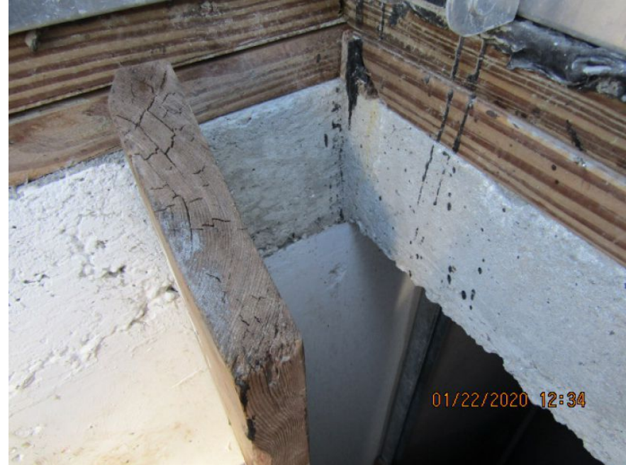
Reinforced Concrete Roof Deck
