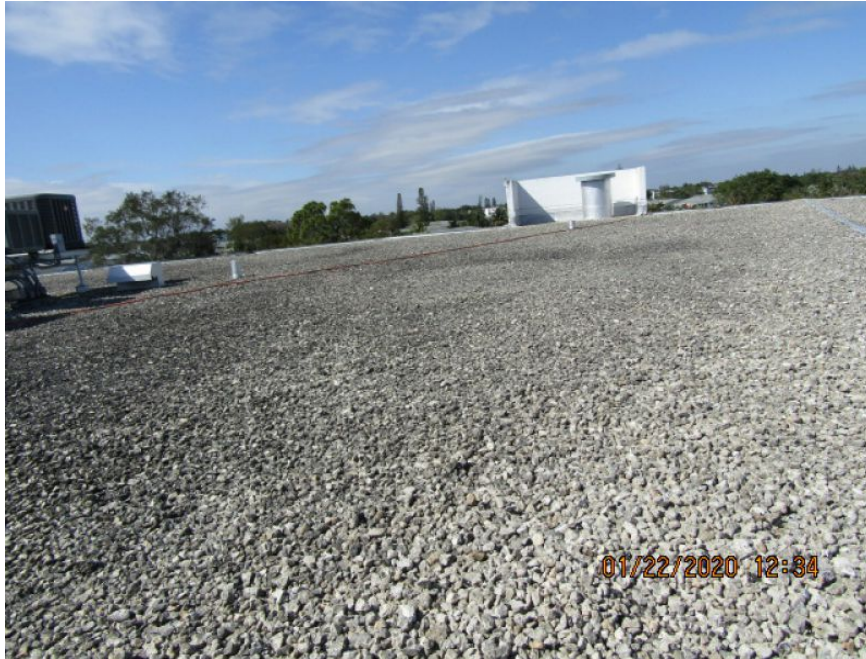
Built-Up Tar & Gravel Roof Covering
