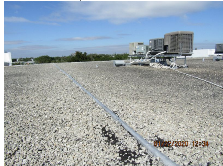
Built-Up Tar & Gravel Roof Covering
